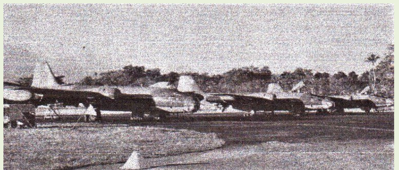
Parking space for three Canberras at Bauer Field
